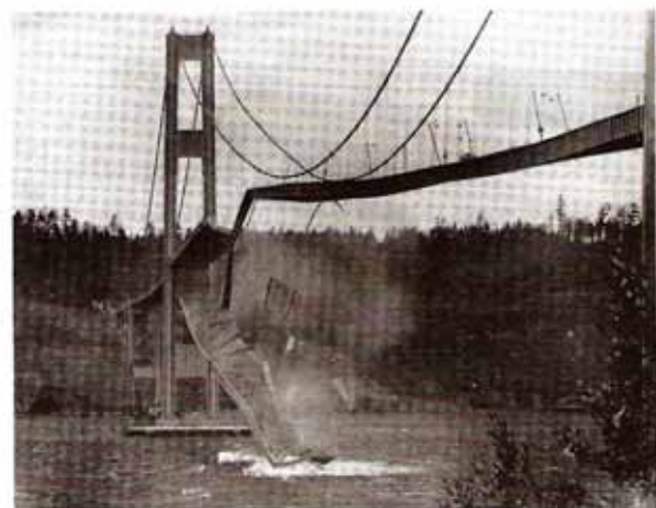
Figure 6.12 The Tacoma Narrows bridge collapsed in 1940, a victim of resonant failure.
