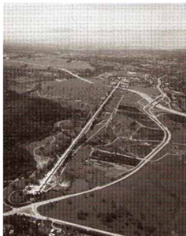
Figure J2.4 An aerial view of the SLAC complex.
